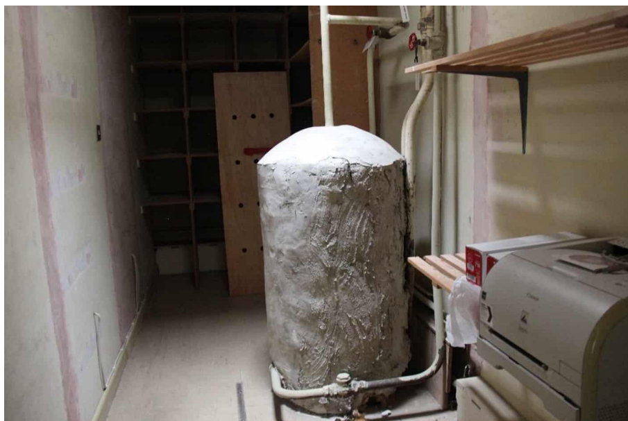
Photograph 59 - One of two walk-in Hot Presses on this level with cementitious layer to water cylinder. May have ACMs.
