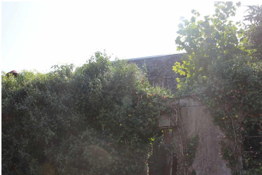
Photograph 3 View of the rear roof plane.
