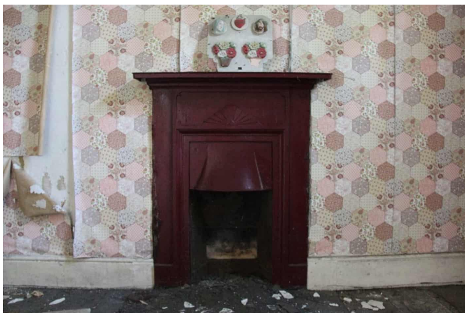
Photograph 24 - Original cast iron fireplace to rear bedroom.
