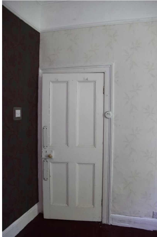
Photograph 46 - Four panel door with brass doorknob.
