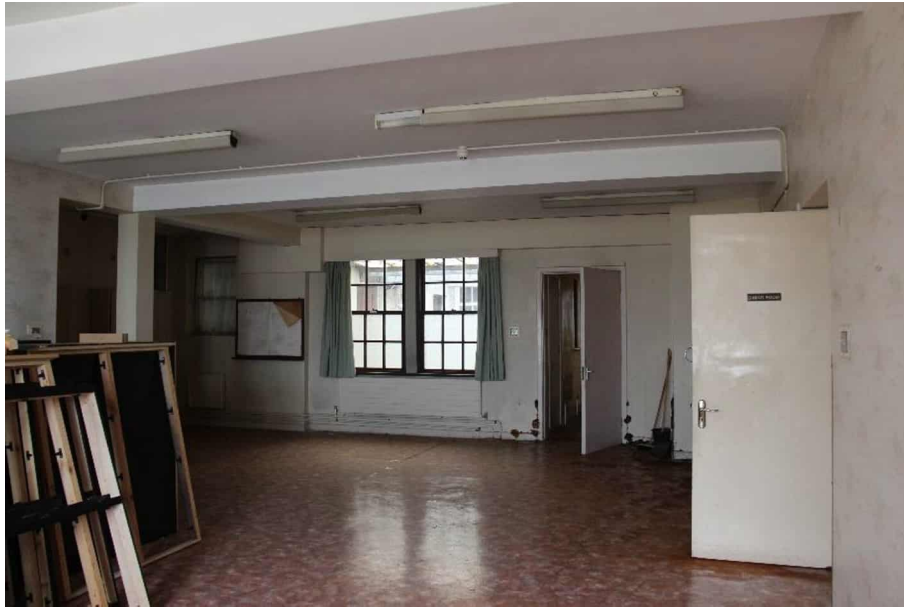
Photograph 18 - modern plasterboard ceiling to later extension.
