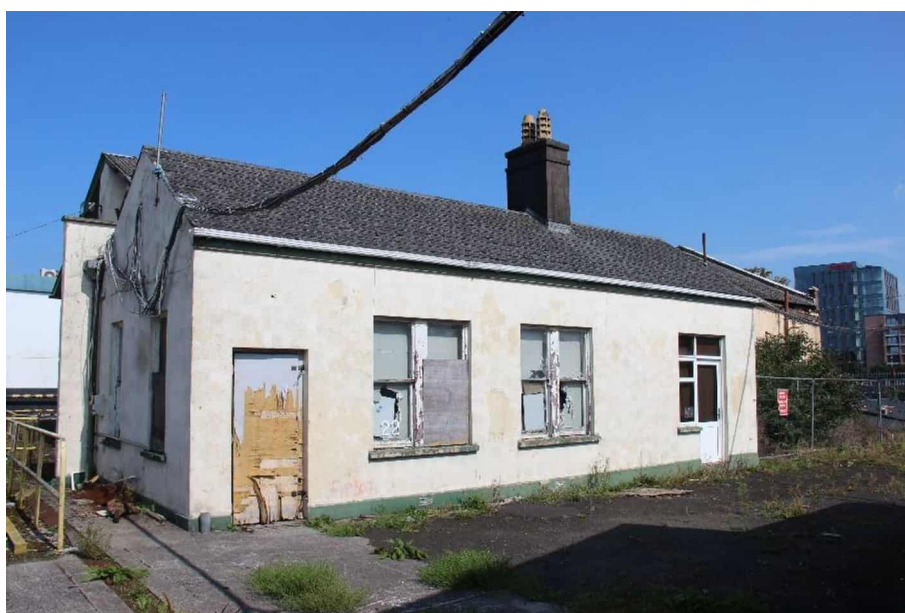
Photograph 3 General view of the “welfare” building.
