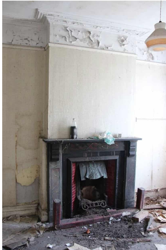
Photograph 13 - Fireplace front room 1st RHS.
