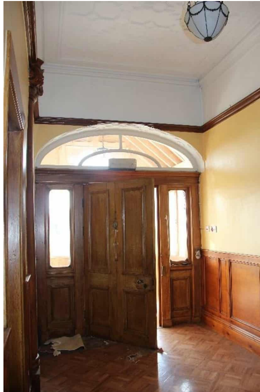
Photograph 14 - Modern ceiling tile to Entrance Hall.
