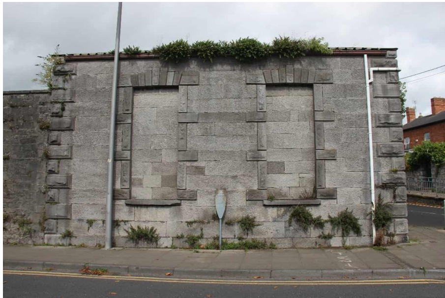
Photograph 1 – Linen Store Southeast Elevation
