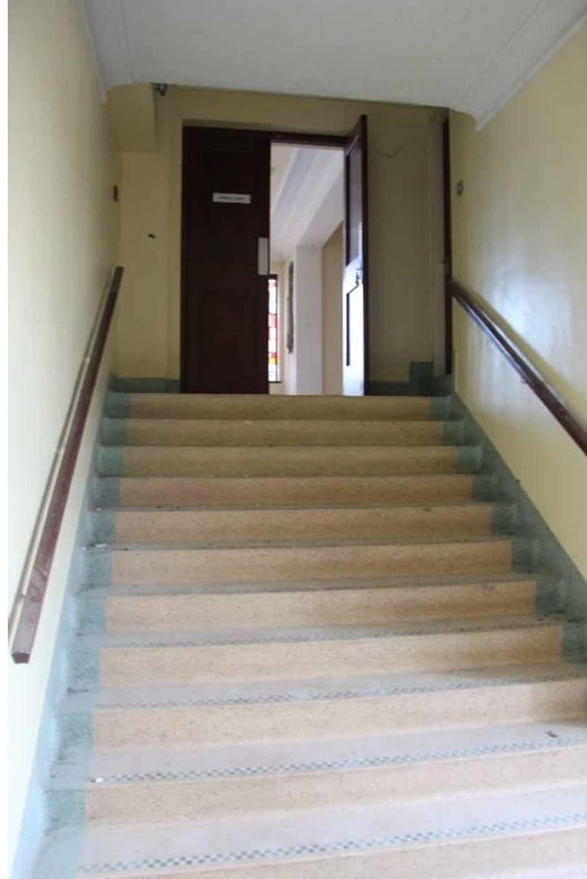
Photograph 47 - modern Terrazzo staircase from chapel to lower level.
