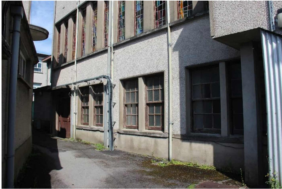
Photograph 13 - Modern timber sliding sash with obscured glazing.
