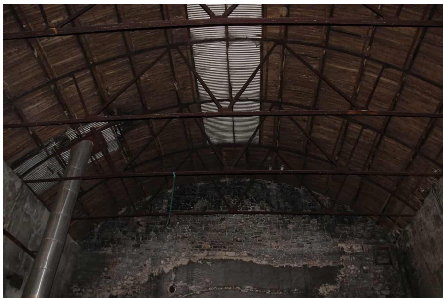
Photograph 12 View of the Roof Build-up of the Engine House.
