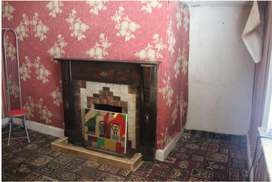
Photograph 37 - Replacement fireplace surround room 1st RHS.
