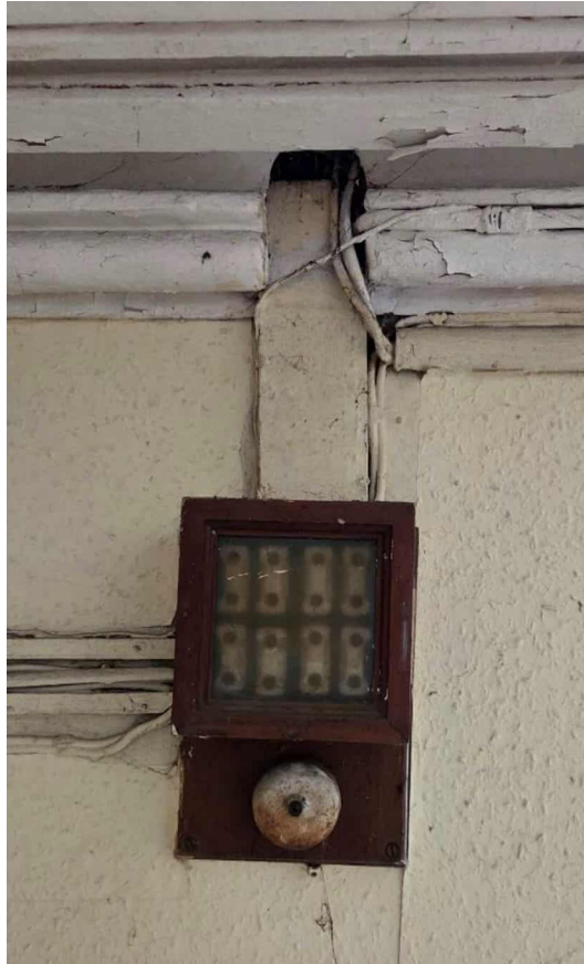
Photograph 16 - Early room service electric bell ring.
