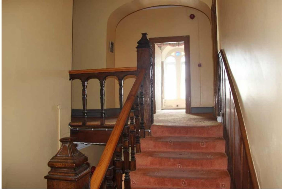
Photograph 45 - Decorative newels and timber wainscoting to first floor landing of original building.
