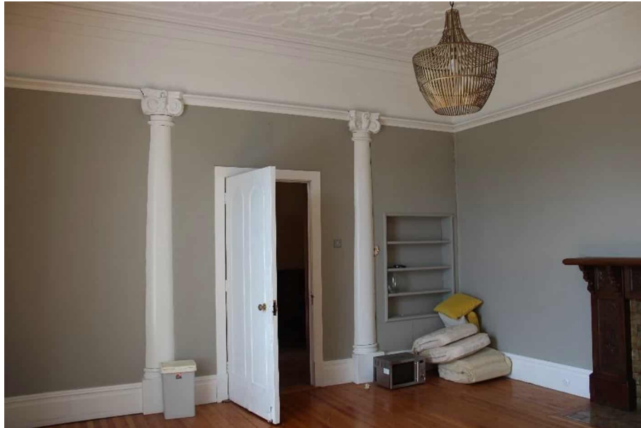
Photograph 20 - Decorative pilasters to partition 1st room RHS.
