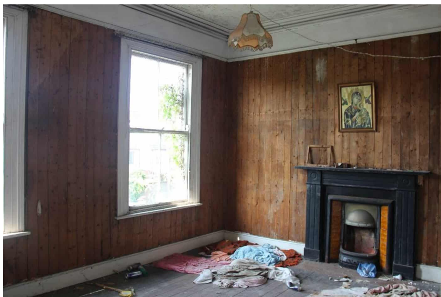
Photograph 23 Front room internal partition and inner face of external wall finished in timber boarding.
